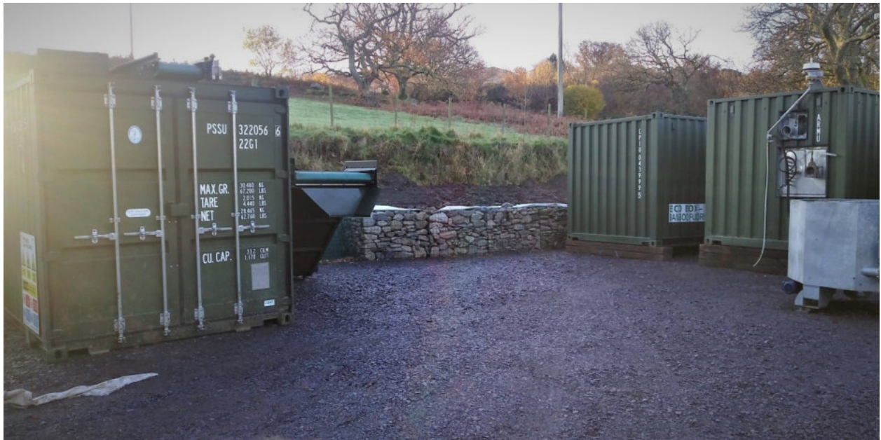
Picture of the IFBB plant placed to the prepared site at Ffarm Moelyci
