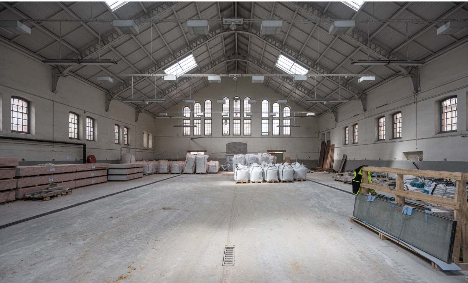
The grand hall, converted into a vast covered storage space for new products and reused components.
