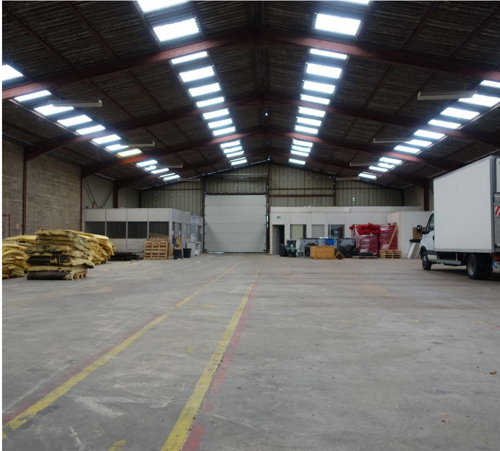
Warehouse view © Rotor
