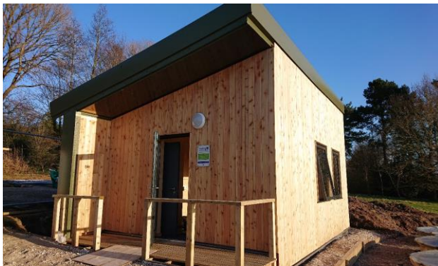
Fig. 1. The UK Demonstrator structure in Ness Gardens, Wirral, Cheshire, UK
