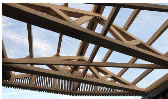
Fig. 7. AF roof truss of the French Demonstrator structure
