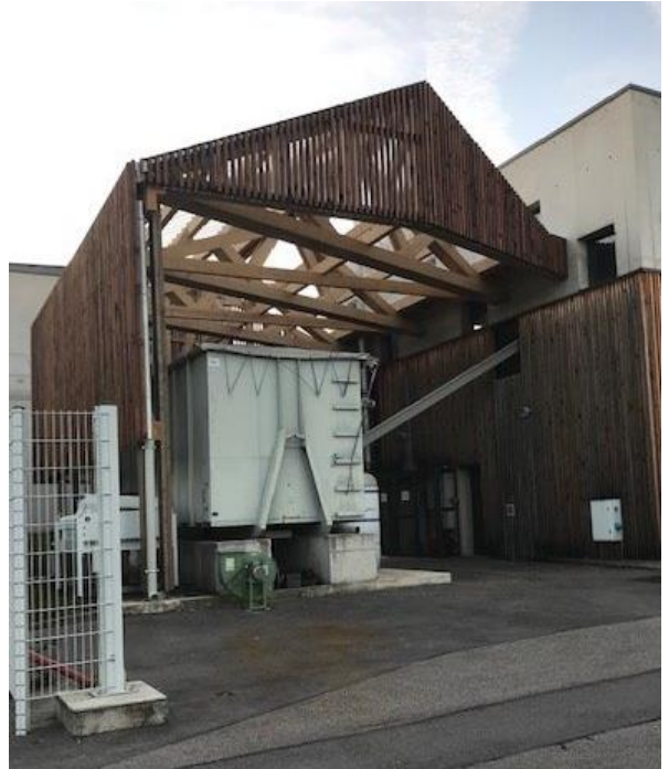
Fig. 8. Completed Structure of the French Demonstrator
