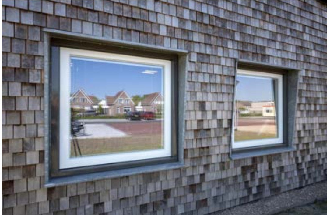
Image source: Rothuizen architecten
