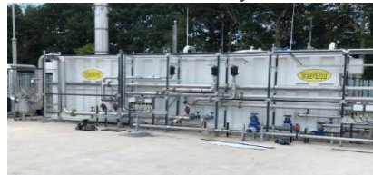
3 polyethylene hollow fibre ultrafiltration membrane registers with a total membrane area of 1074 m 2 ( SFC-Trant )
