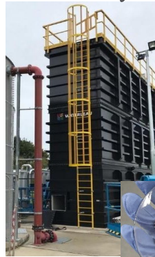
Rectangular 200 m 3 reactor with 6.7 m of water height ( Waterleau )
