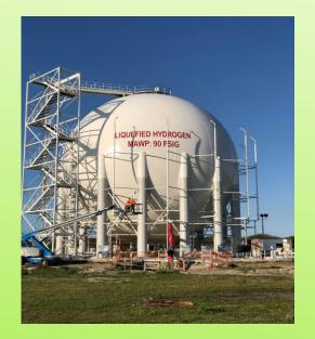
Largest LH2 Tank, NASA Florida Usable capacity = 4,732 m3 **(282,000 kg)** Max. boiloff 0.048% (2,271 L/day) Temp= 4k Pressure= 6 bar
