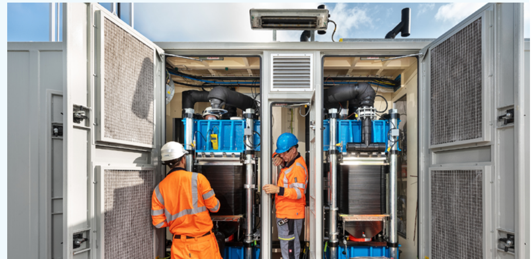
Technicians perform maintenance on a Proton Exchange Membrane (PEM) electrolyzer at a hydrogen energy pilot project inside Gasunie's Hystock site in Veendam, the Netherlands.
